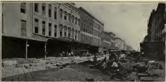
POYDRAS STREET, NEW ORLEANS, IN PROCESS OF REPAIR These heavy granite blocks were relaid as a base for the new pavement
